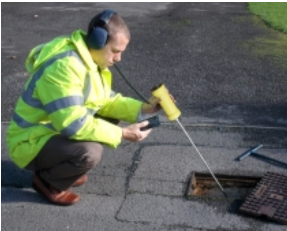
Leak Sizer used for direct leak listening
